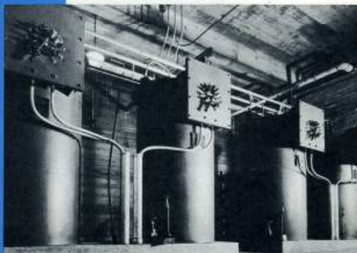
High voltage transformers that step up voltage to supply the plates of the water cooled tubes.
