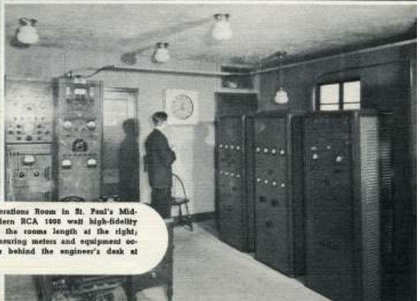
Master Control Room contains amplification equipment for studio operation, control consoles for regulating intensity and "level" of broadcasts and transcribing machines.
